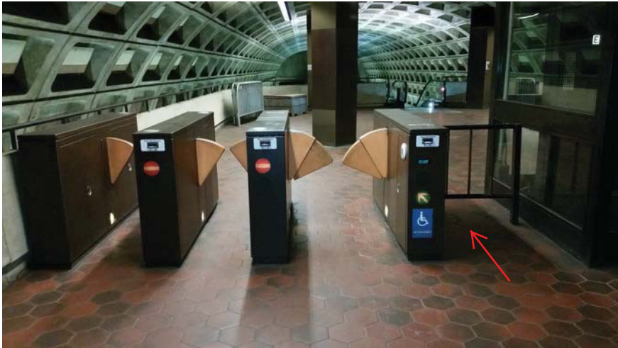
Pictures 2-4: D01 Federal Triangle – Manholes in between both faregate arrays
