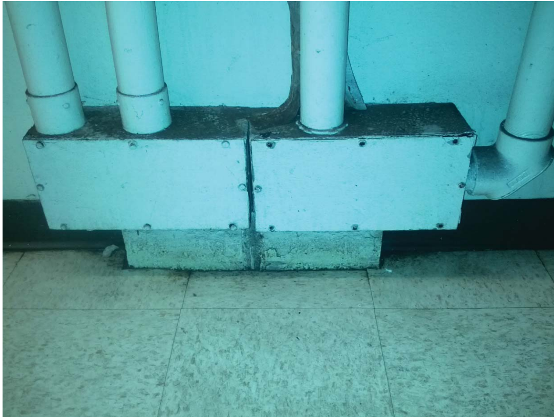
L'Enfant Plaza East Photo #3 – AFC Panel (EF) – Bottom Trough (NOT SHARED) and Walker Duct Transition
