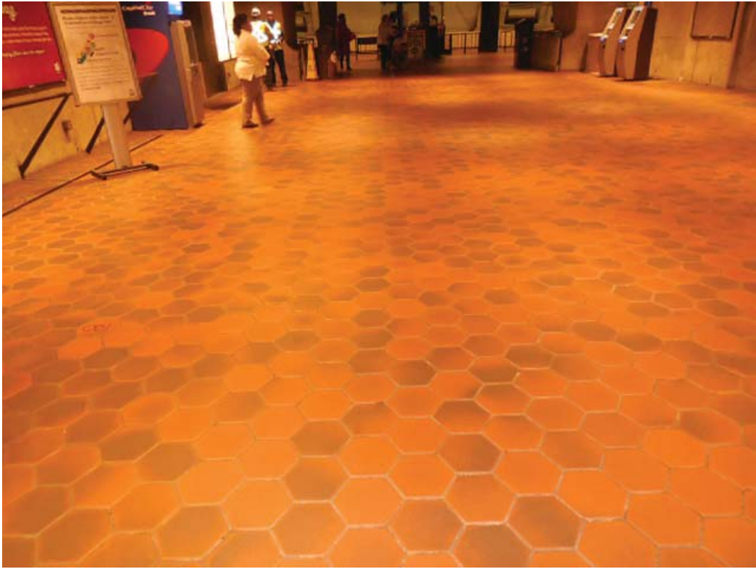
Picture 1: D01 Federal Triangle – No handholes in entrance passageway
