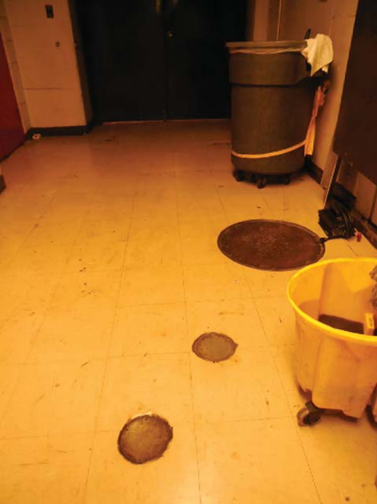
Picture 1: D06 Eastern Market – Manhole & handholes in Service Room
