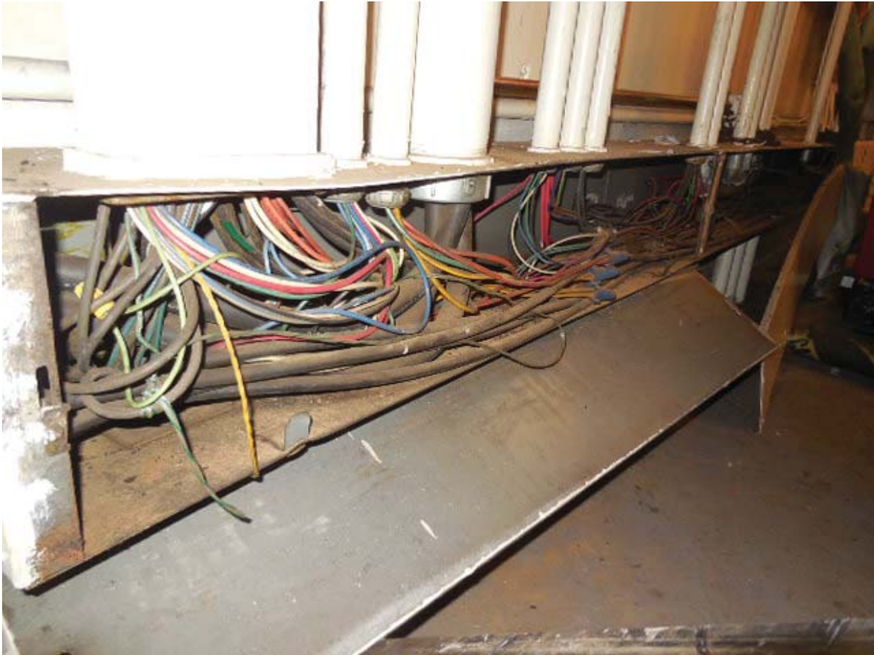
Picture 11: D02 Smithsonian North – Common trough for Panels NM, NM-E, NMH-E, NMH, & NMPO in Room 215
