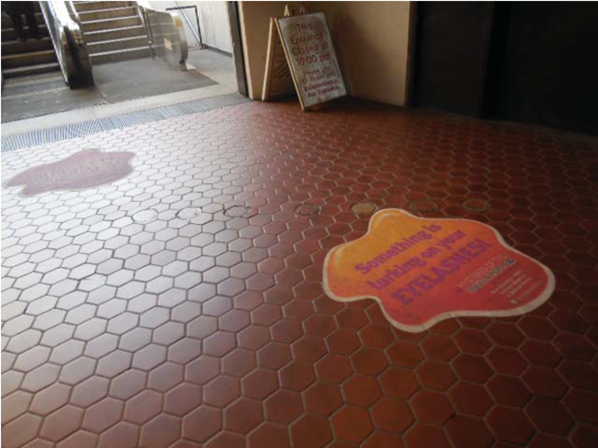
Picture 1: D02 Smithsonian North – Handholes on Mezzanine
