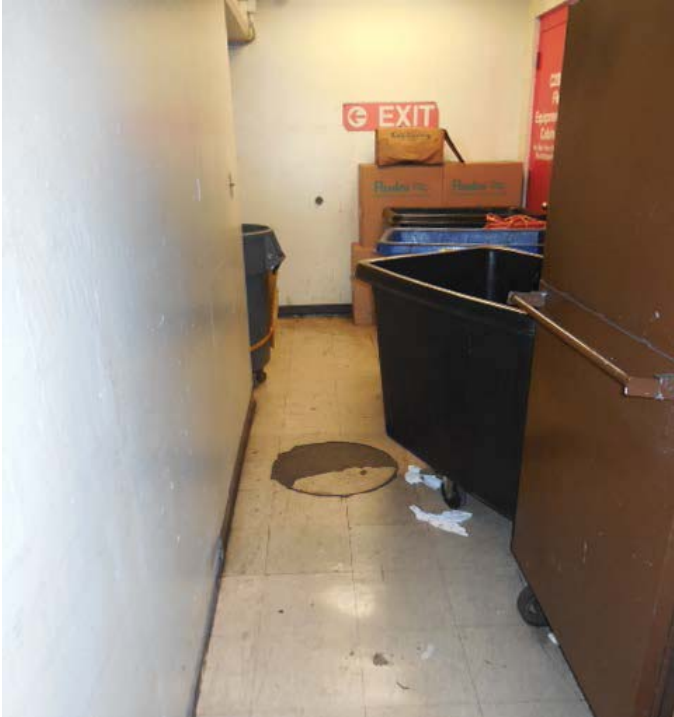
Pictures 3&4: D04 Federal Center SW – Manholes in maintenance corridor
